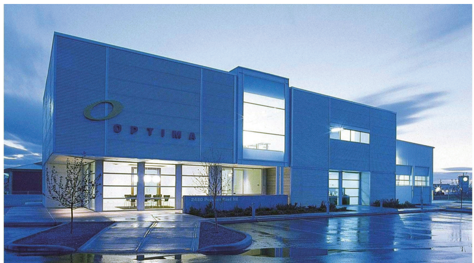
Optima Manufacturing's recently expanded modern facility contains state-of-the-art CNC multi-axis machining centers and turning centers, CNC EDM machines, grinders, and additional machining support equipment.
